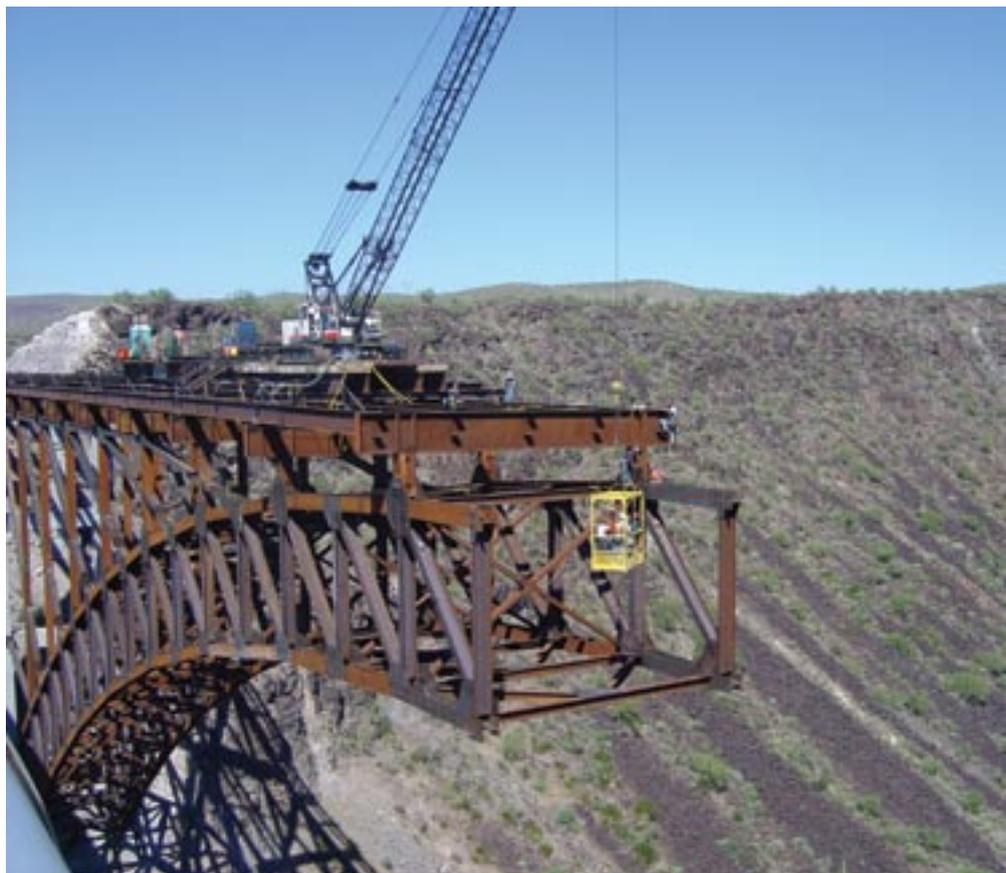
provide support and anchorage for the cantilever launch of the steel arch over the canyon. Flexible connection details were provided for ease of fabrication, transport, and field erection.
