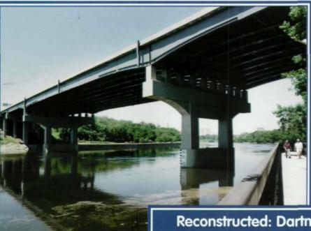
Jurors Comments: "Reconstructed and widened by extending and prestressing the bent caps...a very nice aesthetic iob"
